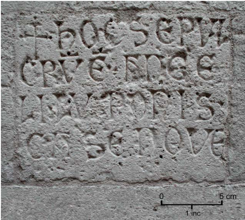
Fig. 26.3. Bari, Apulia, Italy - Funerary inscription walled in the eastern facade of the transept of the Cathedral of Bari, XI-XIII d. C., unpublished: ((cru)) hoc sepul/cru(m) e(st) Ange/li Luponis /Casenove
